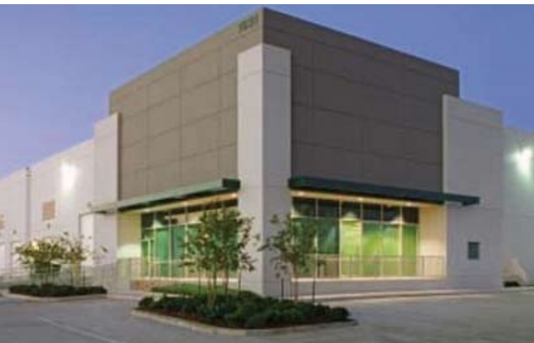
Northstar Commercial Partners recent industrial acquisition - Houston, TX
